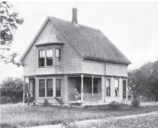
Methodist Protestant Church c.1856 Dismantled in the 1890s and rebuilt as Ridgeway's house Photograph Swann Photo collection CIHS
